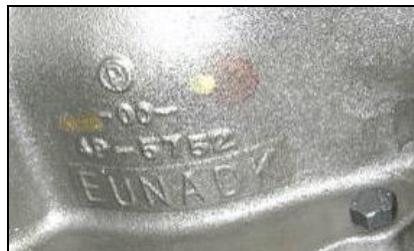
Figure 1 – Typical Foundry / Supplier Identification Marking
