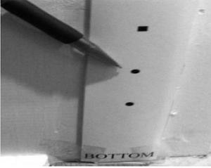
2) Puncture the **BLACK CIRCLES (Figure 2)** and mark with a pencil the 4 screw locations, at the bottom and top of the template, in the center of the circles. Remove the template and where you just marked with pencil drill with 5/64" drill bit a pilot hole for screws **(B)**.
