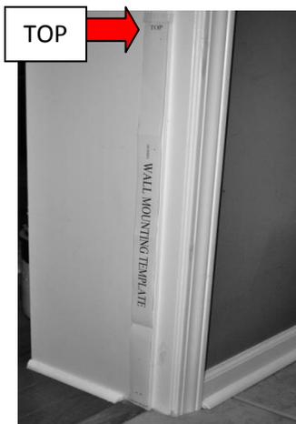
1) Place the mounting template **(A)** vertically on the wall with "Top" on the template located at the top **(Figure 1)**. The bottom of the template **(A)** should be touching the floor (it may be convenient to hold the template in place with masking tape).
