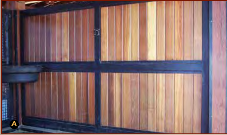
Full wood partition made with 2" x 4" tubular steel for vertical wood.
