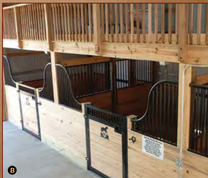
Low rise Kimberwick stall system with wood fill door. Note that the builder omitted the wood channels for a line of seamless fronts.
