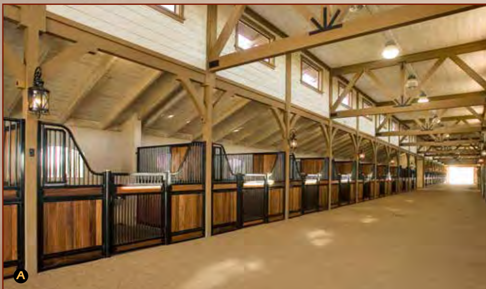
Standard low rise stall front with grill feed door, brass caps and horizontal / vertical wood fill. Hinged grill door with nameplate board and shavings guard.
