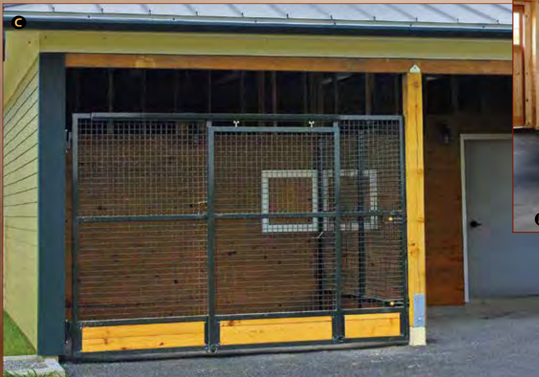
C Full mesh front with offset center doorway and oversized shavings guard. Note that the entire front is hinged to allow easy access for cleaning into this pasture shelter stall.
