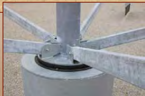
C Fully welded 36" base is made from ¾" steel pipe. The 26" turntable style German bearing rests between the tower and base.
