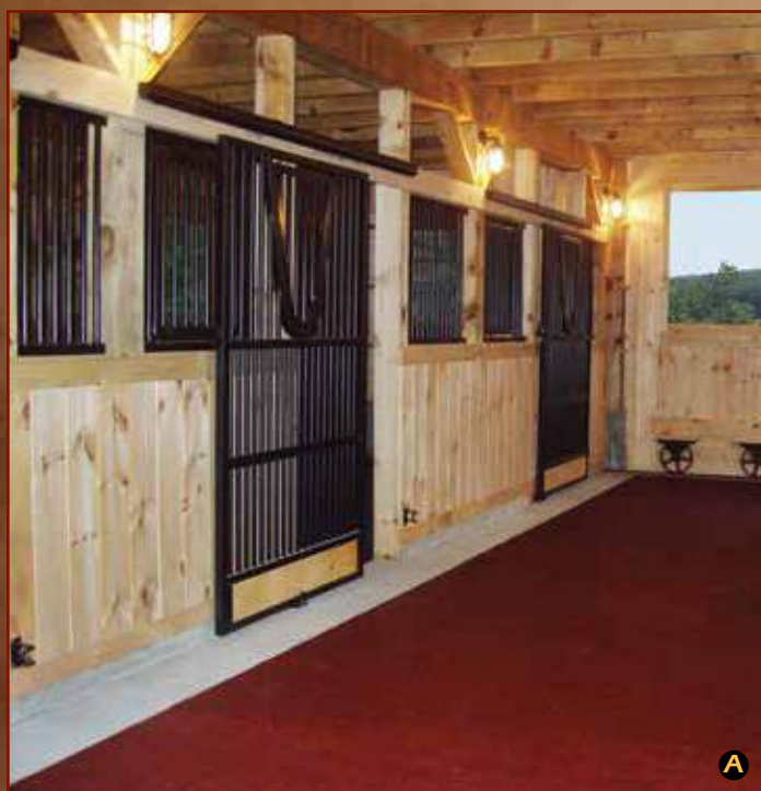
A Center entry stall front with grill feed door. Full grill sliding door with yoke opening, removable fill piece and shavings guard.
