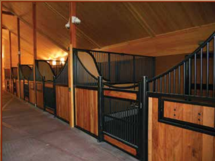
A Low Arc stall front with painted caps. Hinged grill door with nameplate board; shavings guard. Note custom partitions with radiused privacy section.
