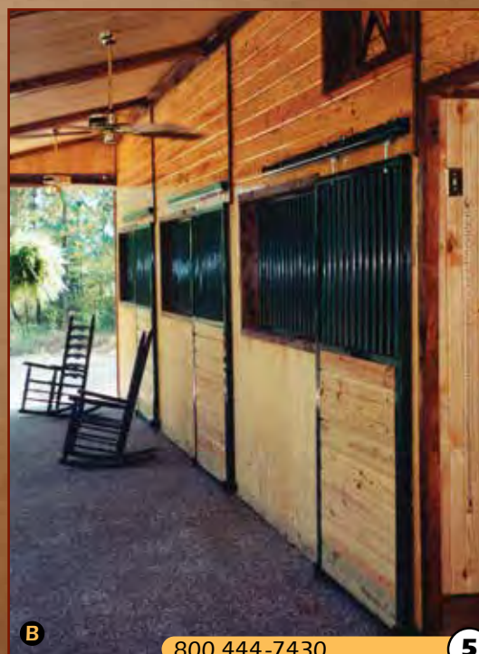
B Side entry stall front with feed opening. Sliding door with grill top and horizontal wood fill bottom.
