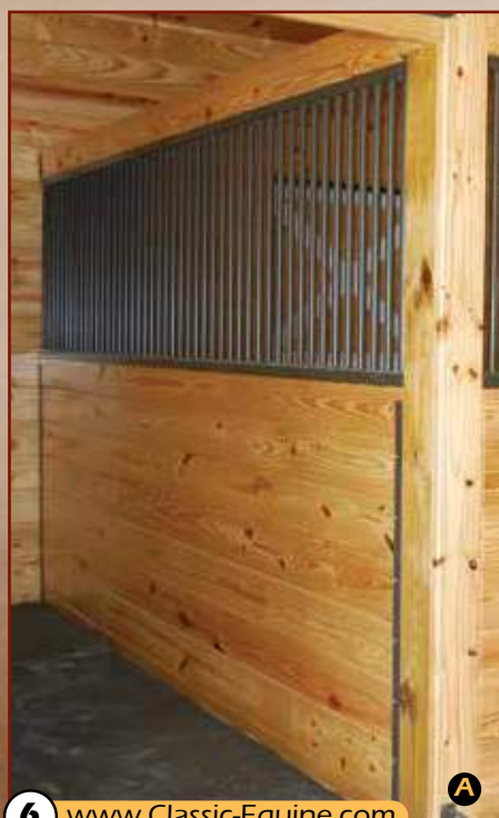
A 12' partition grillwork with 48" U-channel for bottom horizontal wood.
