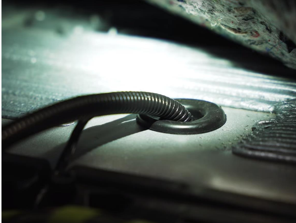
Photo of wiring harness being routed into the cab of the vehicle through the floorboard.
